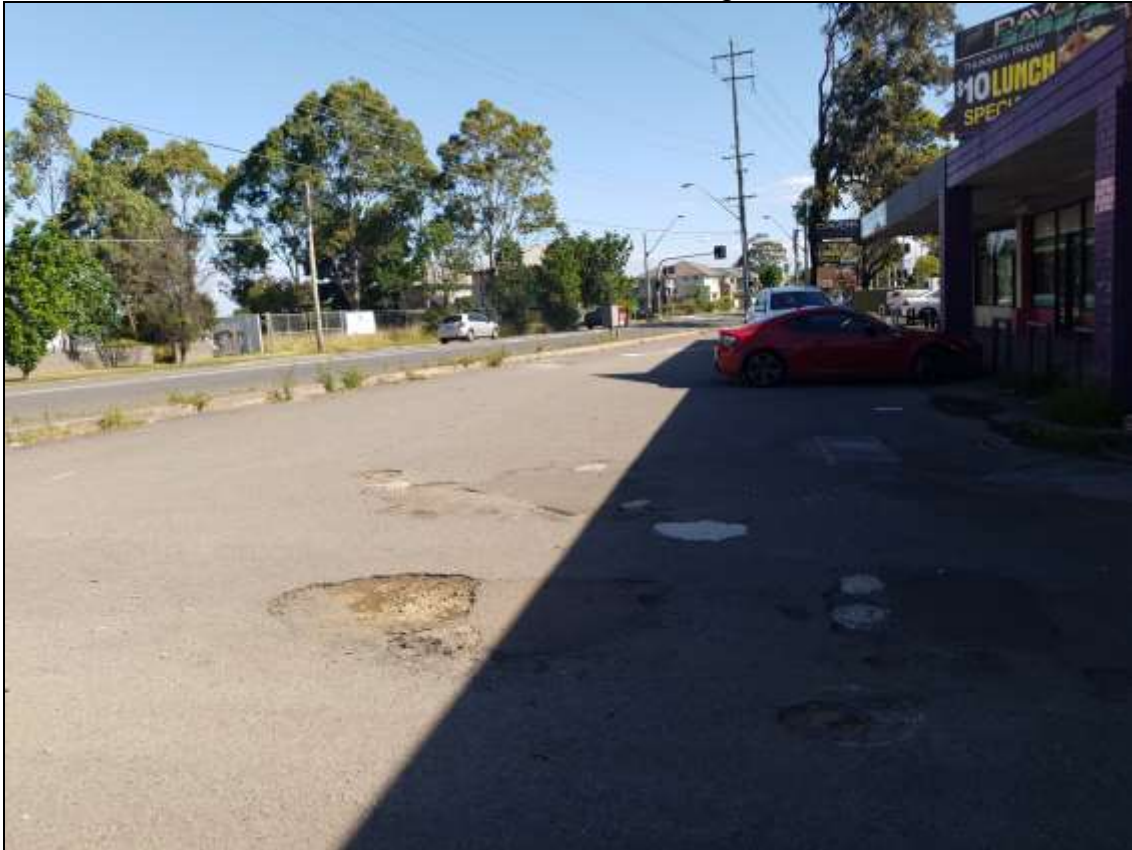
Front Car Park, Cracked and Damaged Pavement
